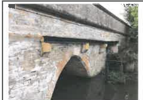
FIGURE 10 – GENERAL VIEW OF STEEL JOIST AND STONE CORBEL
