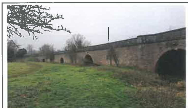
FIGURE 1 – VIEW OF OUNDLE NORTH BRIDGE
